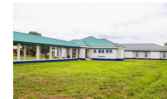
Built, Furnished and Commissioned Amenity Ward at Kwale, Delta State
